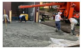
our loading dock was completed in August. A crew from Ellis Concrete took up the old concrete and replaced it with a fresh 6-
